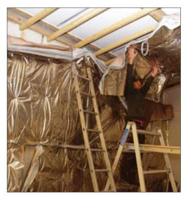
insulation and avoidance of thermal bridges.
